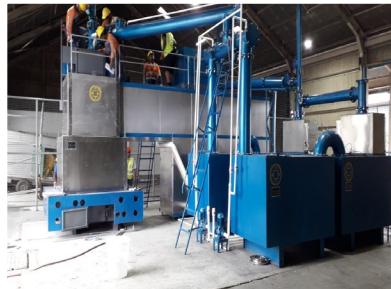
Installation of an Electric Incinerator to meet international requirements
