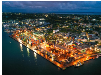
Upgrading of facilities with energy-efficient LED lighting
