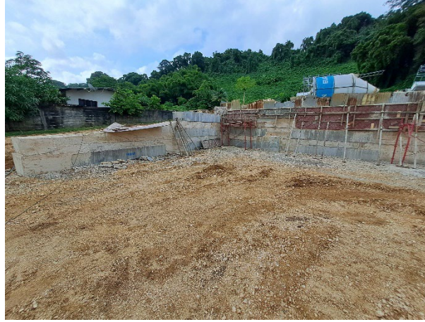
Reuse of old beams in mass retaining wall
