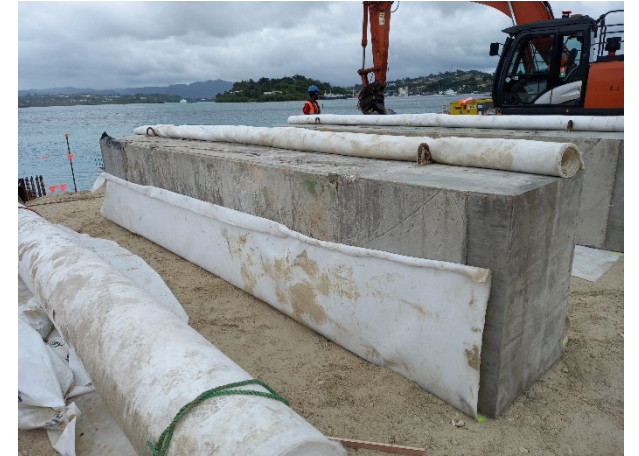
Upcycled precast for revetment toe
