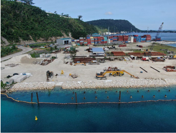
Re-use of old rock armour in sheltered locations
